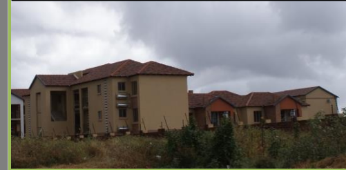
2-3 Storey Medium Density Development
